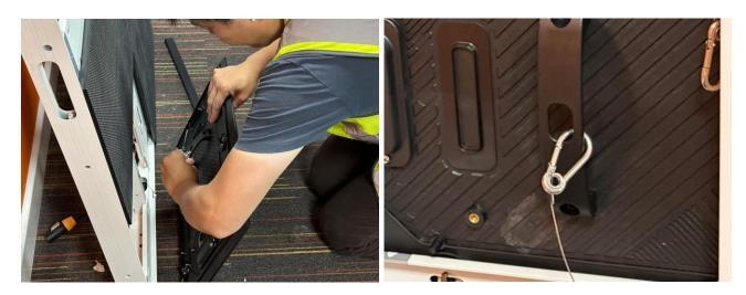
**Step 5**Mount the DV-LED cabinet to the rails using the Unistrut Long Spring Channel Nuts. Ensure you tighten the bolts to secure the cabinet to the rails.
