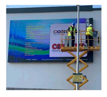
Our installation team managed the install, working alongside a local partner. The lightweight LED cabinet structure, as well as the magnetic modules and positioning pins, ensured a smooth installation.
